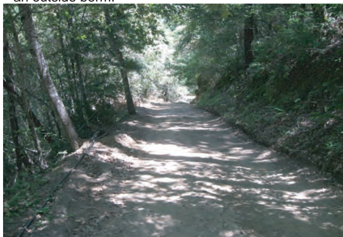
Midslope portion of undrained driveway that contains an outside berm.
