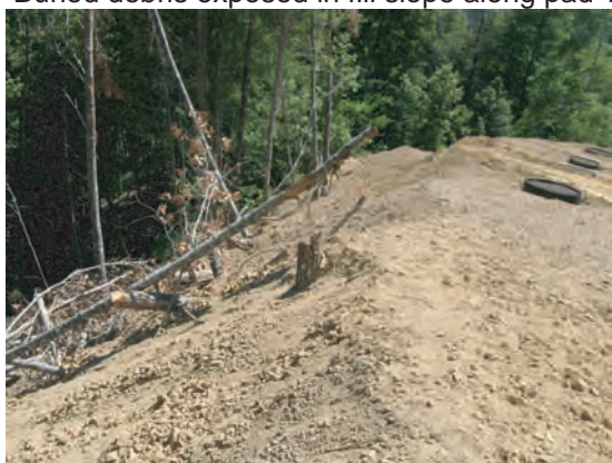
Debris exposed in fill slope along pad 1.
