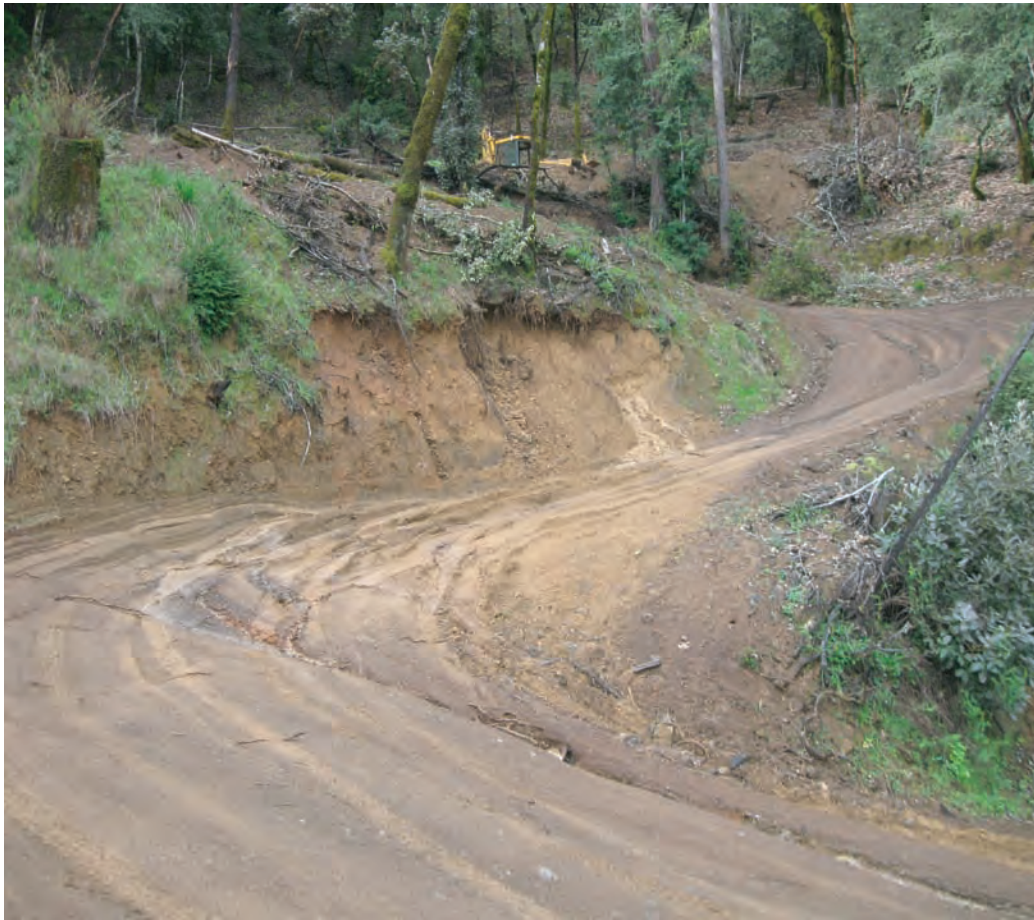
Photograph 3. Erosion on existing unpaved access road, 1111 Doolan Canyon Drive. Photograph by CGS, March 3, 2010.
